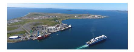
Port of Argentia is a premier heavy industrial seaport offering ice-free, year-round access, a wide turning basin, heavy lift capacity, and up to 11-metre draught alongside 430 metres of dock facilities at the Argentia Marine Terminal.
